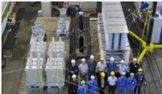
Mitsubishi Electric DCCB testing
