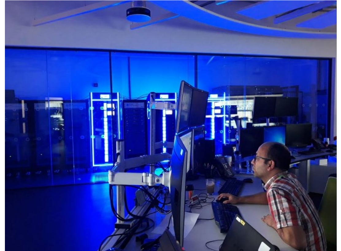
Source: National HVDC Centre (UK)
