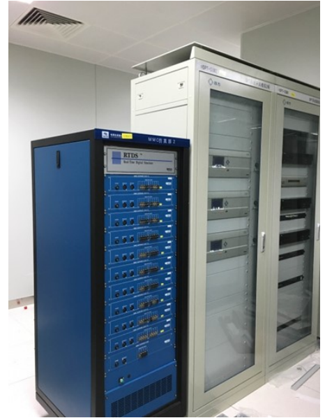
Control and protection cubicle alongside the RTDS Simulator's GTFPGA Units for MMC simulation
