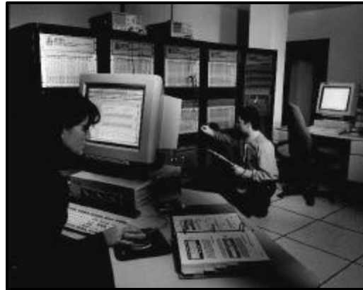
Fig. 1 RTDS Simulator Installation
