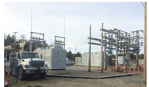
Installation of skidmount transformers at BC Hydro's remote Masset substation on Haida Gwaii. Transformer protection was tested with the RTDS Simulator.
