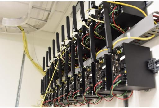
Figure 10 – Communication infrastructure with 23 RX1400 Modems
