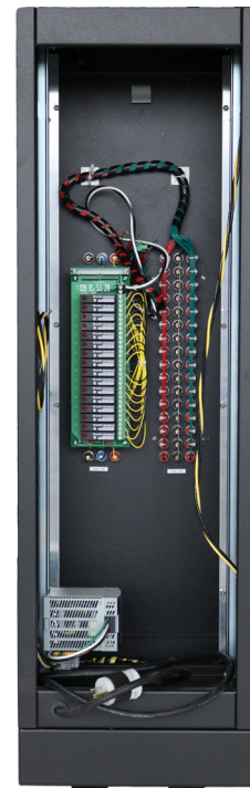
Additional I/O cards and power supplies are accessible from the rear of the portable I/O cubicle
